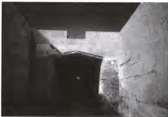
Fig. 2-4. The Ostrian "third" temple at Abydos. Top of the wall is at ground level.
